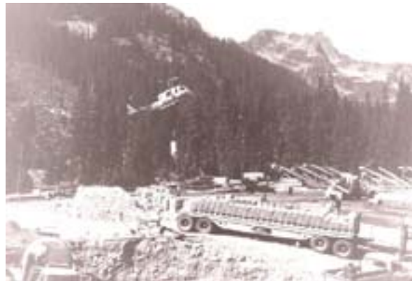
Concrete for lift tower footings.
